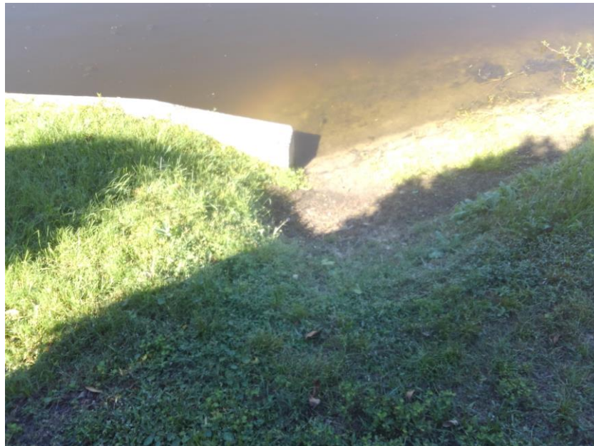
8) Pond 3- Second view of partial soil loss behind drainage structure headwall at south end of pond.
