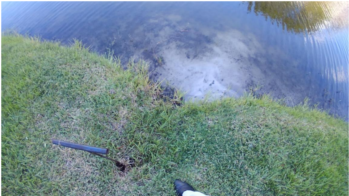
6) Pond 2- Close-up view of depression on pond bank at west side of pond.
