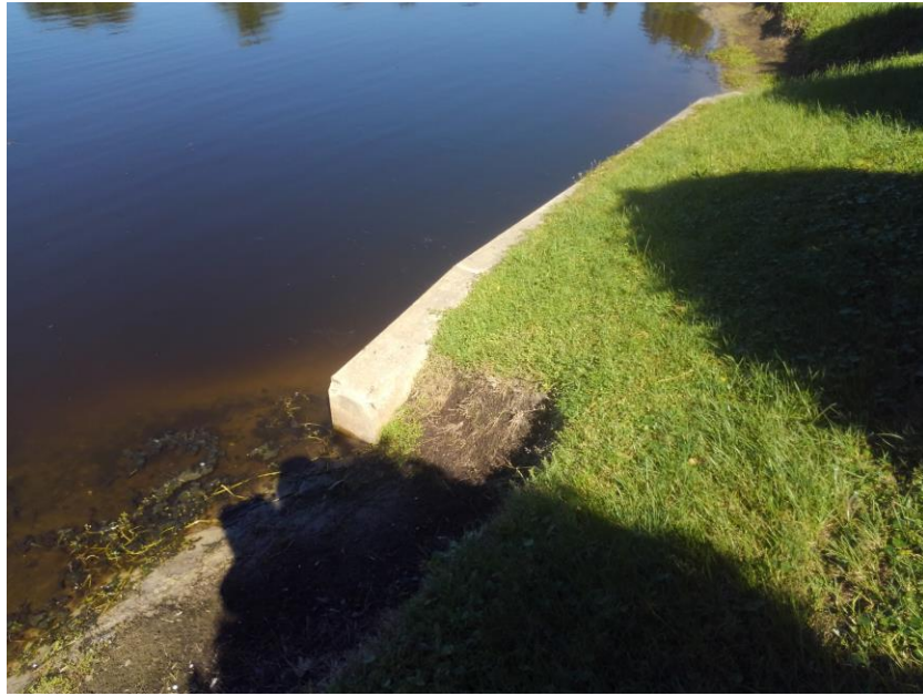
7) Pond 3- Partial soil loss behind drainage structure headwall at south end of pond.
