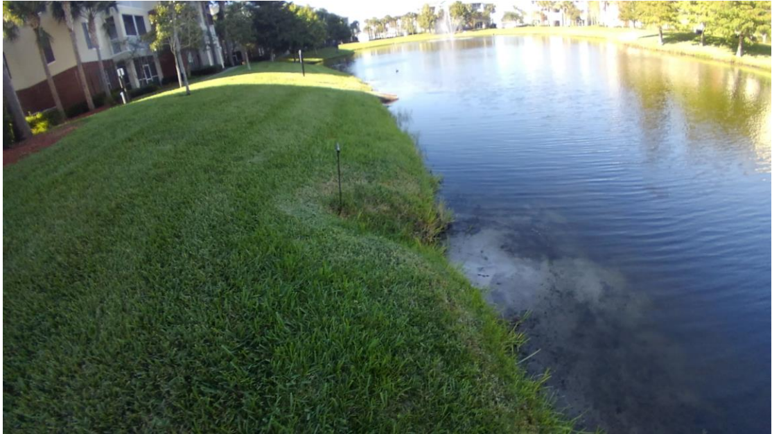
5) Pond 2- Depression on pond bank at west side of pond.
