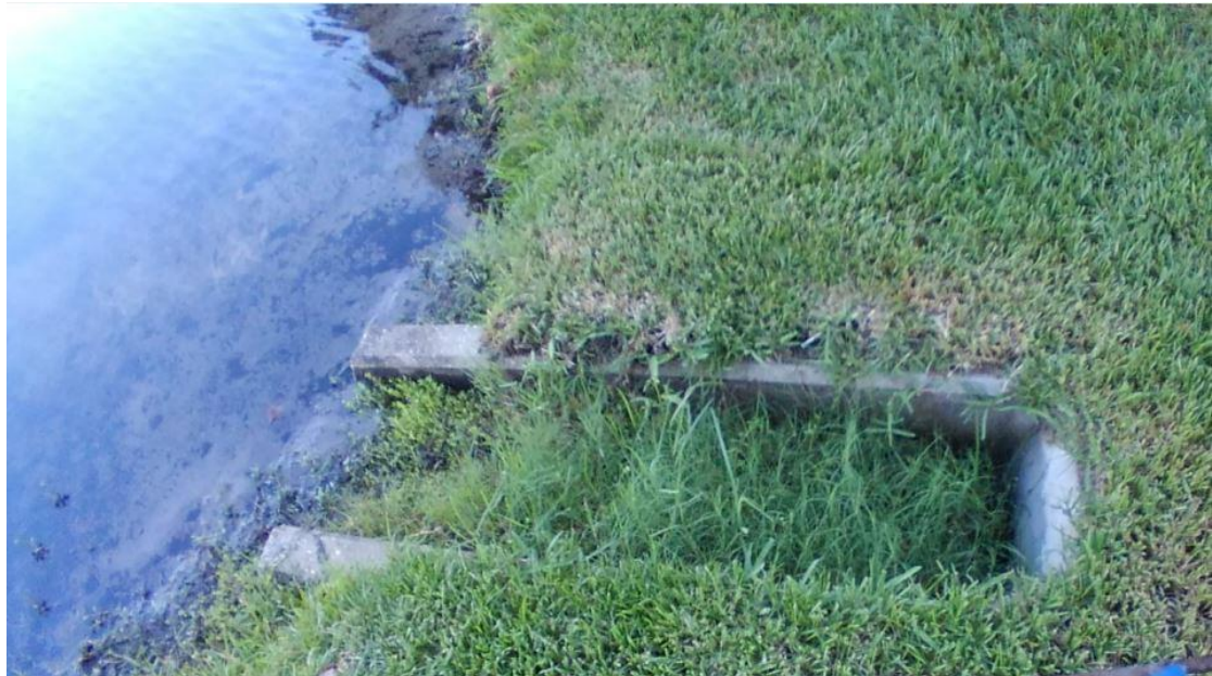
4) Pond 2- View of vegetation partly obstructing drainage at MES drainage structure.
