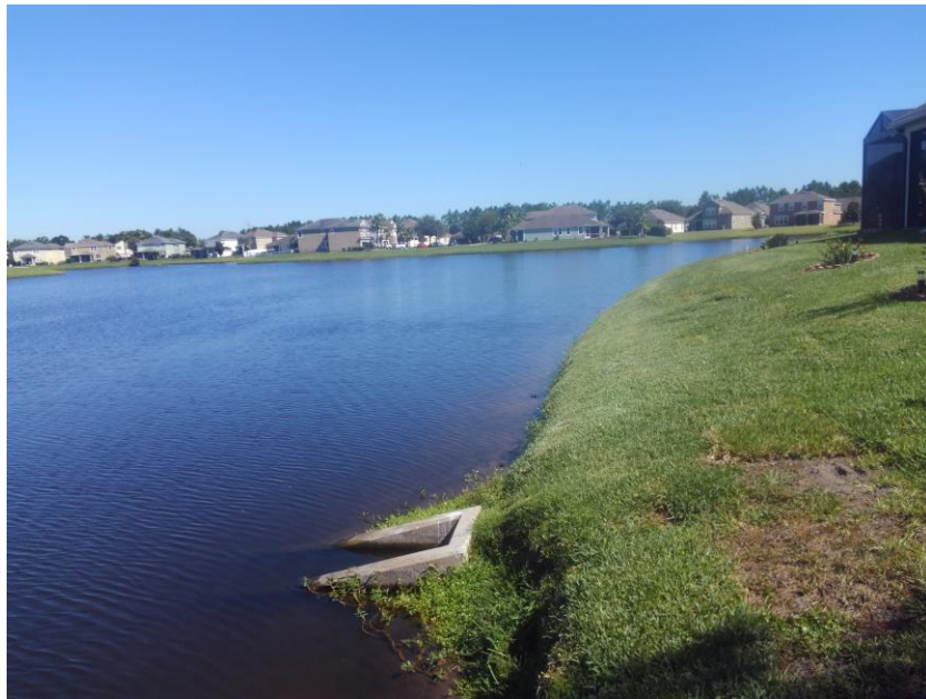
6) Pond 5- Apparent erosion at drainage mitered end section structure between Lots 252 and 253.
