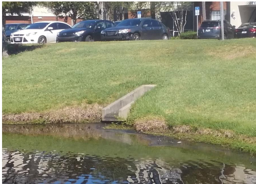
2) Pond 3- Loss of soil/undermined drainage MES structure at east-central portion of pond bank.
