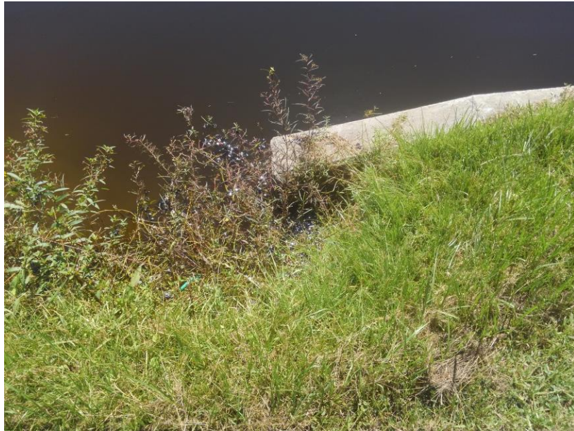
7) Pond 5- Partial loss of soil behind drainage structure headwall.
