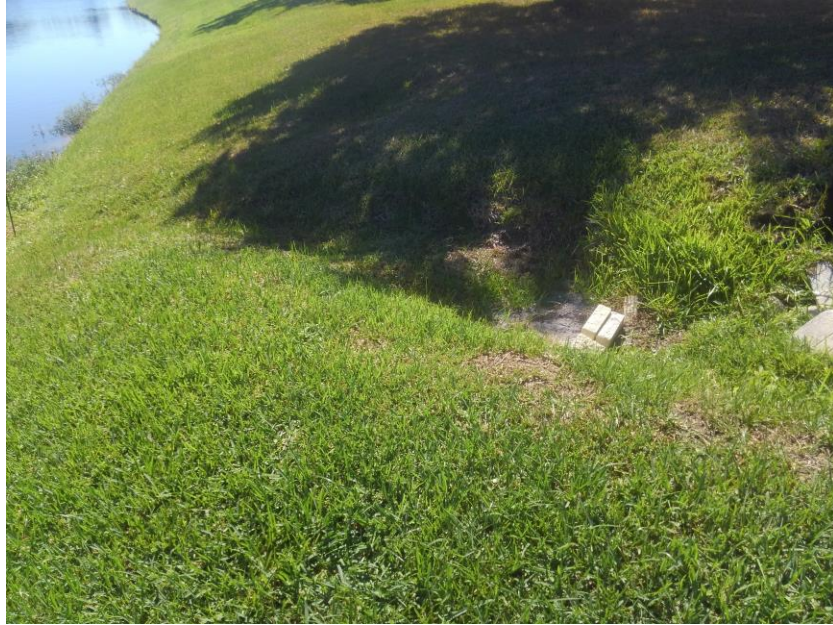
1) Pond 5- View of erosion channel at the pond bank between Lots 284 and 285.
