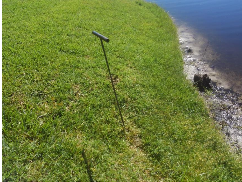
1) Pond 3- Small depression on east side of pond bank.
